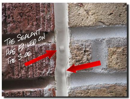
When stretched, the tape will de-bond and create weak points in the joint. It is difficult not to stretch the tape during install...care must be taken.
