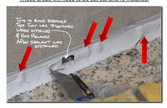
Also, as discussed before, make sure that the <u>correct width</u> tape is installed and allow sufficient time for out-gassing of any ground material underneath!
